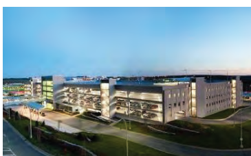
Imp Building Halifax Airport, NS
