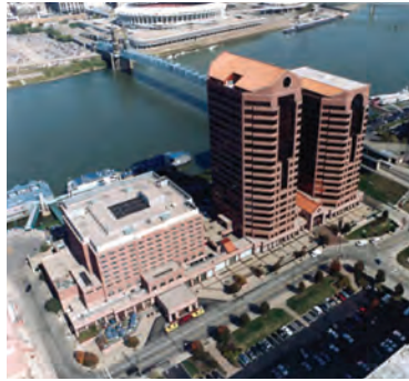
River Center Ofc. Building, Cincinnati, OH
