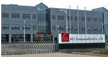
Owens Corning (Hangzhou), Zhejiang
